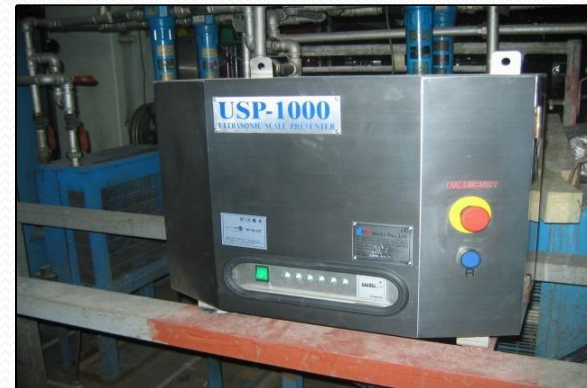
Tancheon Sewage Treatment Plant
