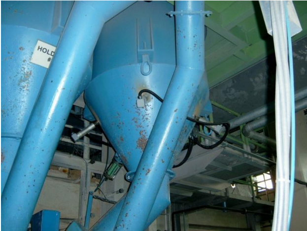
Installing USP to Hopper
