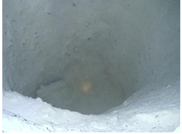
Inside of #4 hold bin before installation
